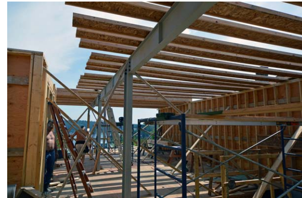
But Most Popular in Home construction Engineered I Beams
