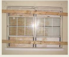
In a good amount of cases, with double hung windows, both windows will be moved to center and the cross brace places above and below. This way when the board up is removed, the windows will be completely operational.
