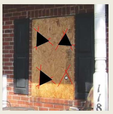
As stared earlier, all cuts can be made but 1, prepping for immediate removed once the call for their removal is made – without delay.
