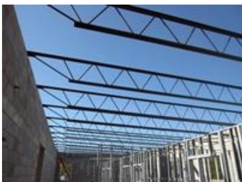
Bar Truss used in supporting both Floors and Roofs
