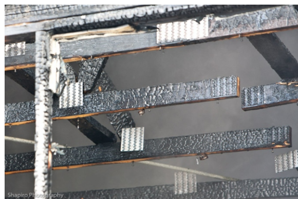
Truss failure due to fire (alligator wood)
