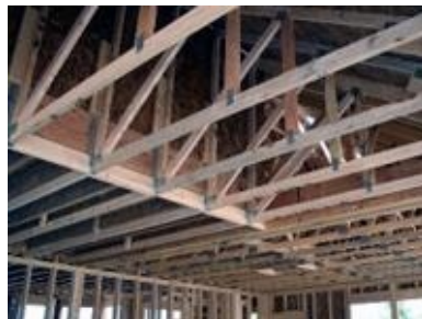
Wood Roof Truss
