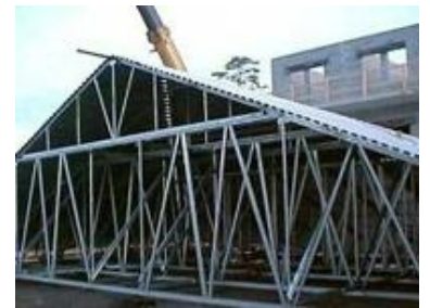
Metal Roof Truss
