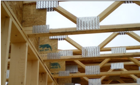
Gusset plate holding 2"x4" truss system together
