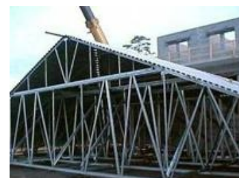
Metal Roof Truss
