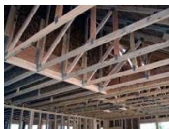
Wood Roof Truss
